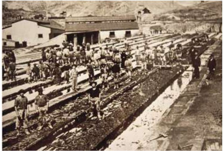
Figure 3.10: Channel system in the Riotinto mines for copper cementation in the first half of the 20th century (Riotinto Foundation).
