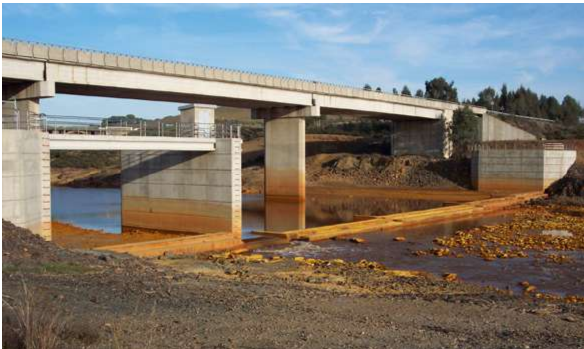
Figure 4.53: Gauge station in the Tinto River at its lower reach (Gadea).
