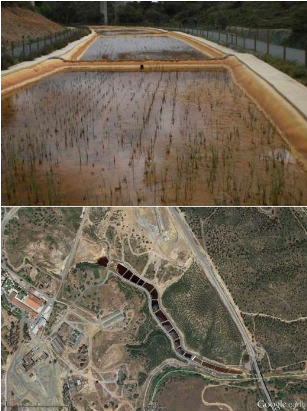
Figure 7.15: Photo and aerial image of an aerobic wetland constructed in Lousal mine (Portugal), with working problems due to the high metal contents of AMD.
