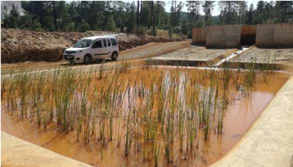
Figure 7.30: Spontaneous appearance of Typha domingensis (cattail) in settling pond 1, demonstrating the significant improvement in the water quality.
