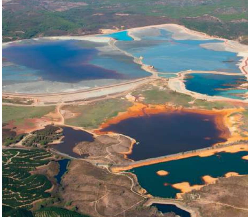
Figure 3.13: Gossan and Copper tailing dams from the Riotinto mines built in the 1970s and currently being raised to store waste from the new operation.
