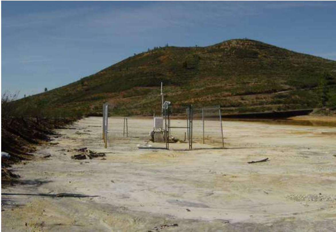
Figure 2.7: Tailings dam in Cueva de la Mora mine, where an experimental station to investigate sulfide oxidation processes was installed in 2008. This dam was subsequently restored and is currently sealed with impermeable materials.
