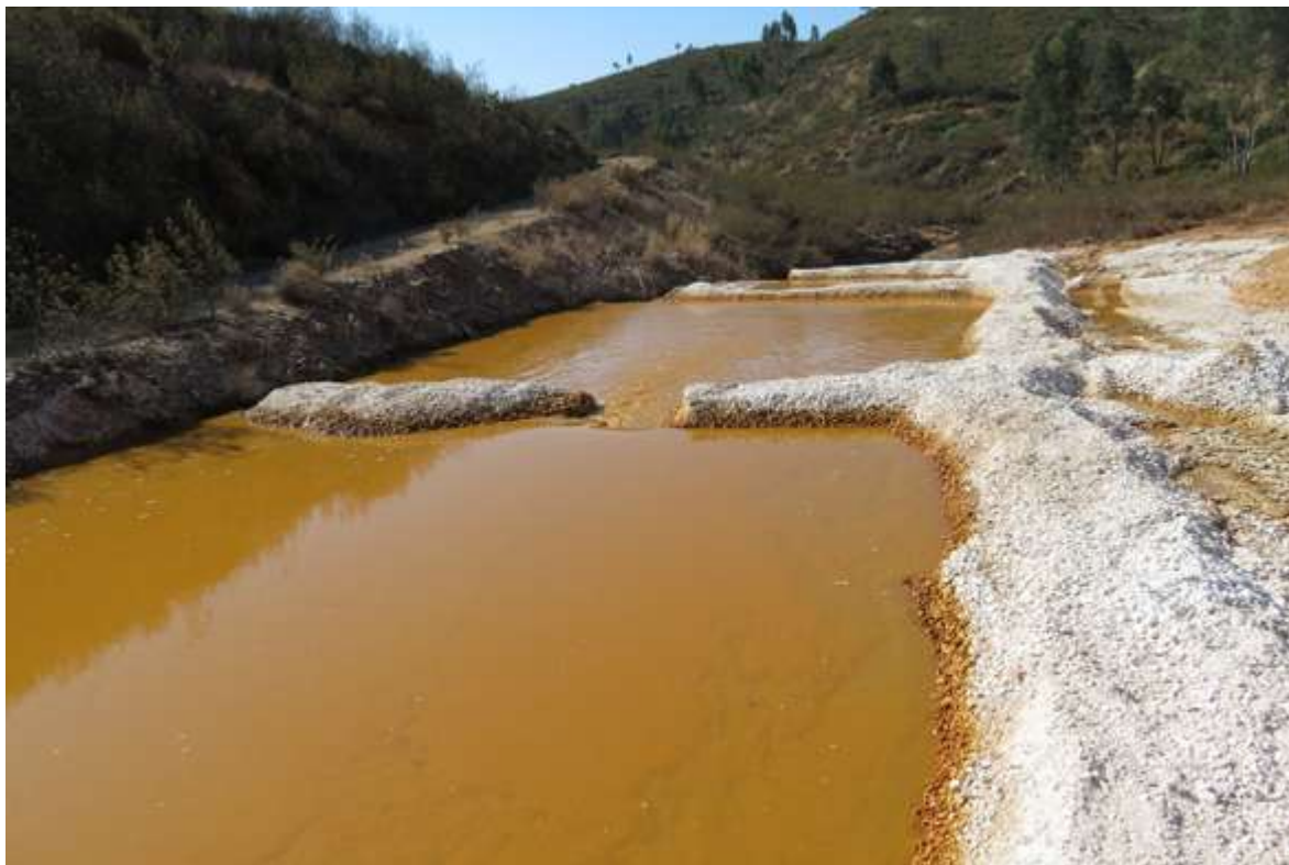
Figure 4.49: Addition of limestone gravel to treat the AMD delivered from the La Zarza spill (May 2017).
