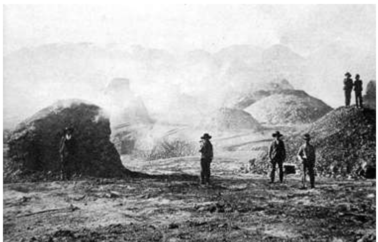
Figure 3.11: "Teleras" (mineral piles) for open-air pyrite roasting during the second half of XIX century (Riotinto Foundation).
