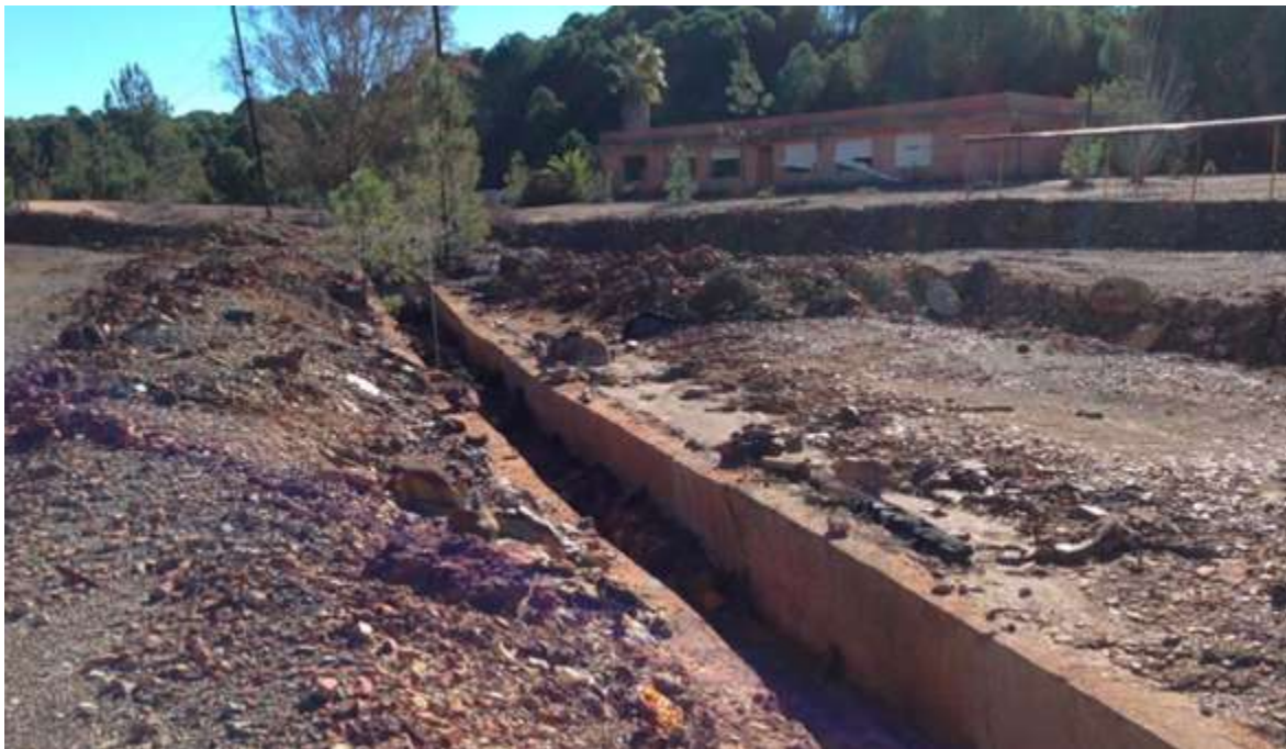
Figure 7.4: Photo of perimeter channel in the Riotinto mines.
