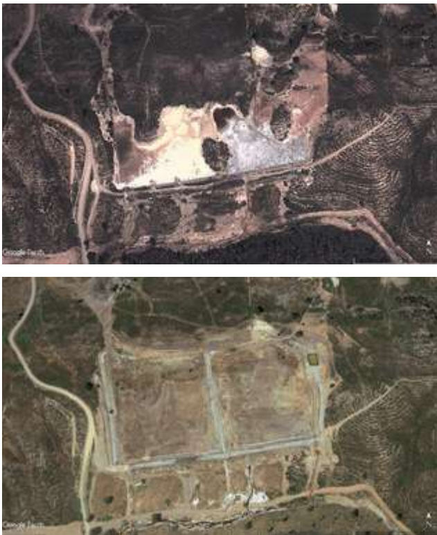
Figure 7.8: Aerial images of tailings dams in Monte Romero mine, previously to the installation. (above, June 2009) and after the implementation of a dry cover (below, July 2013).
