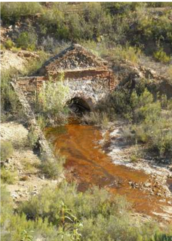
Figure 4.47: Acidic leachates outflowing from Los Cepos gallery before the La Zarza spill (September 2011).
