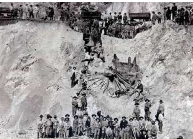
Figure 3.9: Roman-era waterwheel for water extraction in underground mining operations found in the Riotinto mines (Riotinto Foundation).
