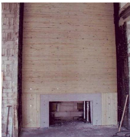
Figure 4.9. Test rig with X-lam layer and concrete window frame
