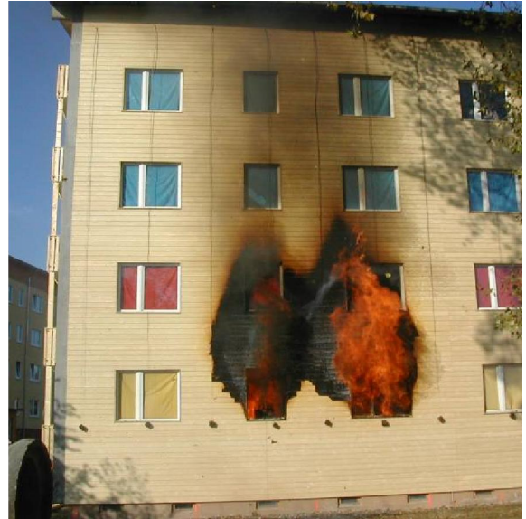
Figure 4.14. Fire in a room next to the exterior wall
