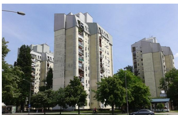
Figure 1 – High-rise residential buildings Type 13
