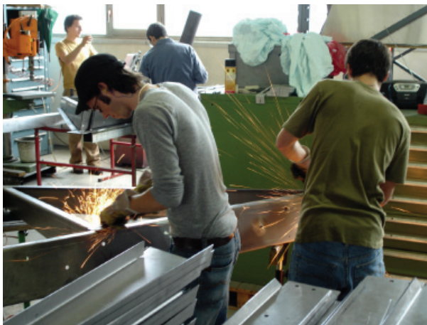
Fig. 1 Students 1:1 METAL WORKS welding the roof. Font: D-ARCH / ETHZ / Deplazes, A Archive (2006)
