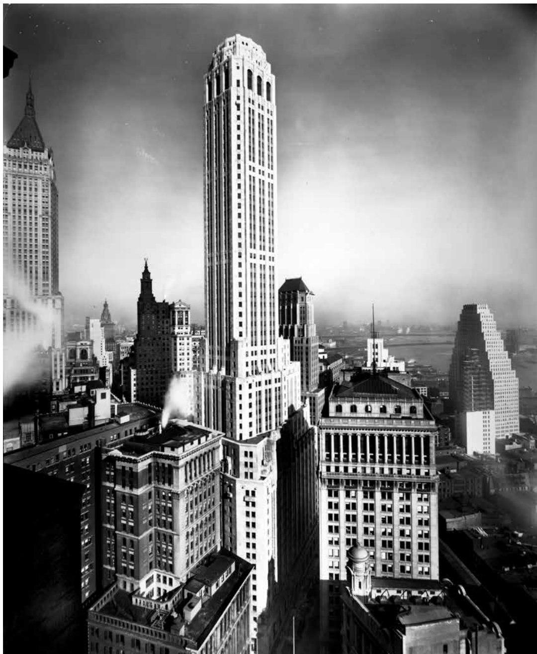
Fig. 55. City Bank Farmers Trust Company Building.
