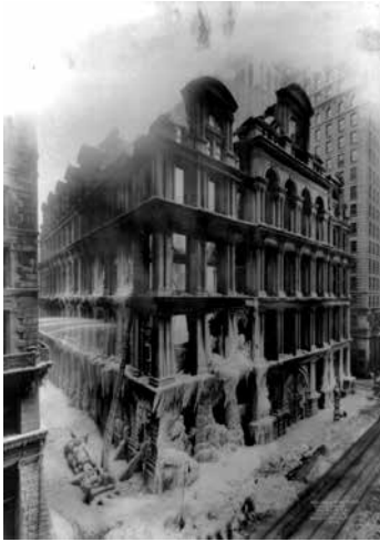
Fig. 36. El incendio del Equitable Life Assurance Building.
