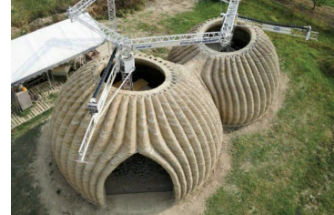
Figure 6. Tecla House, 3D printed on-site using clay by WASP (2021)
