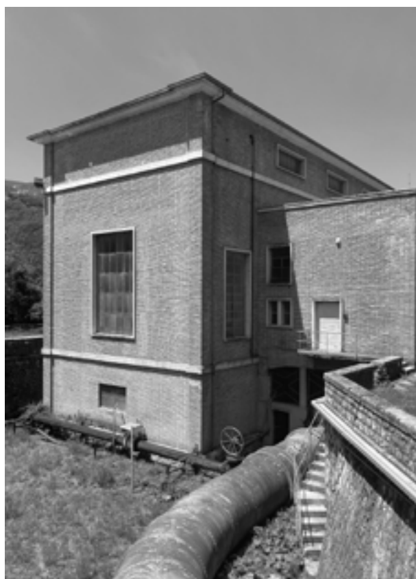
Figure 3. Hydroelectric power plant owned by Burgo Group, in Canistro (AQ).
