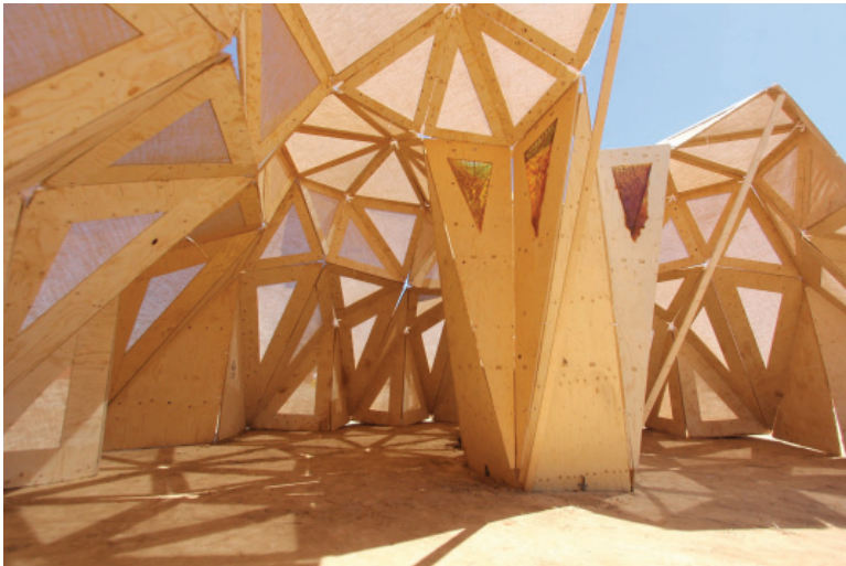
Fig. 3 Nomad Folding Flax Pavilion erected in the desert of Monegros, Zaragoza. Photo by Ji Won Jun (2017)
