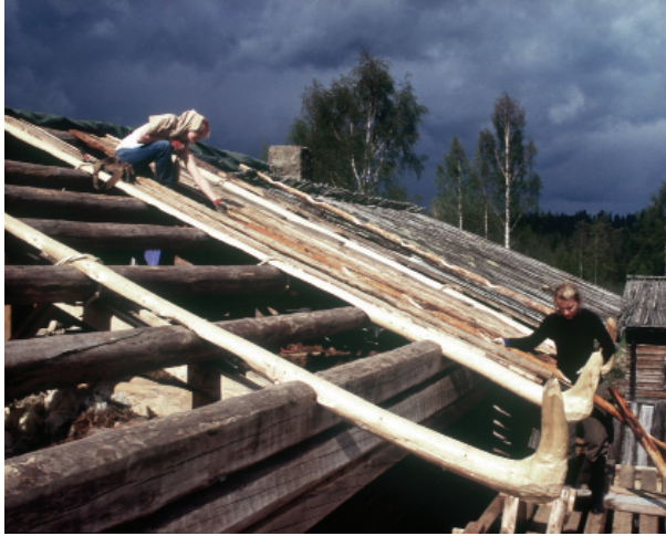
Fig. 3 Aalto University architecture students repairing the roof a wooden house in Murtovaara (2008) using traditional building techniques (photo: courtesy of KSS, Netta Böök, Marko Huttunen, Katja Savolainen)
